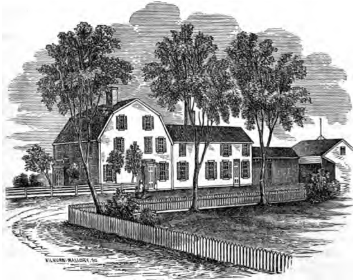
"The Gambrel Roof," as the Bradley mansion is sometimes called, is well represented by the above cut. It was built by Hon.
